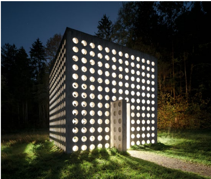
St. Arbogast Water Castle, Götzis | AT Architecture: Christian Lenz, Artist: Fridolin Welte
